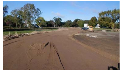
Step #5 - Virtually no stakes at this point
